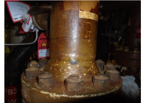
Initial condition of pipework
