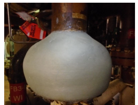
Final cured repair
