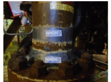
After surface preparation
